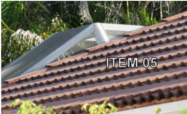
Before: Roof Replacement
