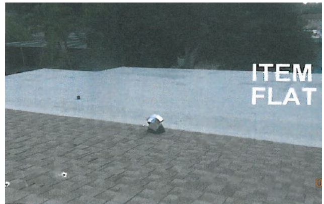
After: Flat Roof Replacement
