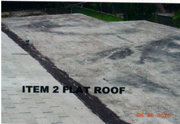
Before: Flat Roof Replacement
