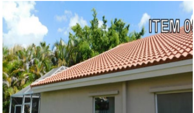
After : Roof Replacement
