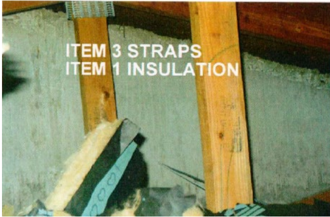
Before: No Insulation
