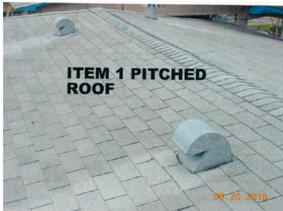
Before: Pitched Roof
