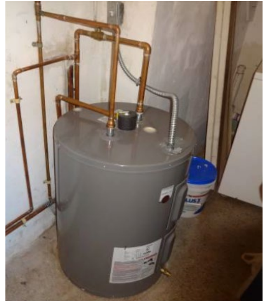
After: Hot Water Heater
