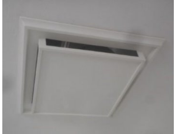
After: Upgraded Exhaust Fan
