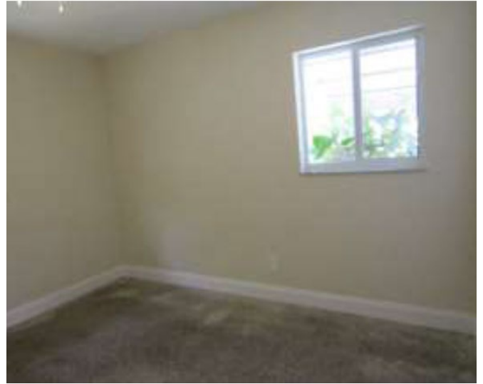
After: New Drywall and Mold Remediation
